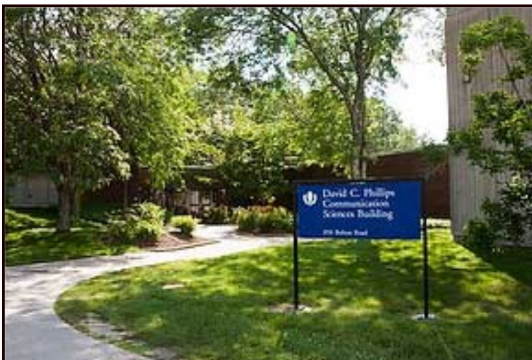
Phillips Communication Sciences Building, home of the Speech and Hearing Clinic at the University of Connecticut © 2021 UConn
